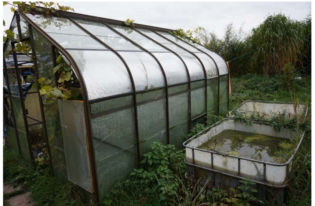
The north side of the greenhouse is protected with insulation so the heat remains inside. As well there is water tanks inside the greenhouse to keep thermal mass.
