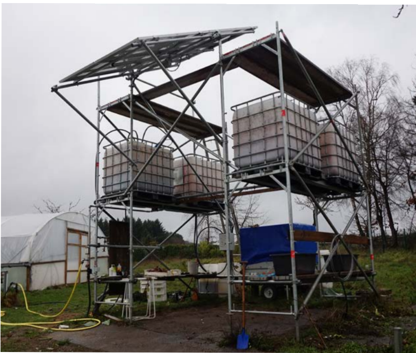
The water tower has sun pannels to pump the rainwater from the greenhouse roofs into the high storage tank and compost tea tanks.
